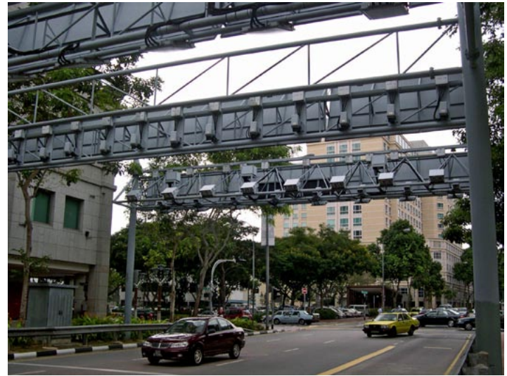
Figure 66 Short-range radio communication system is used to deduct ERP charges automatically.
