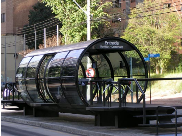
Figure 54 ▲ Bus station in Curitiba.
