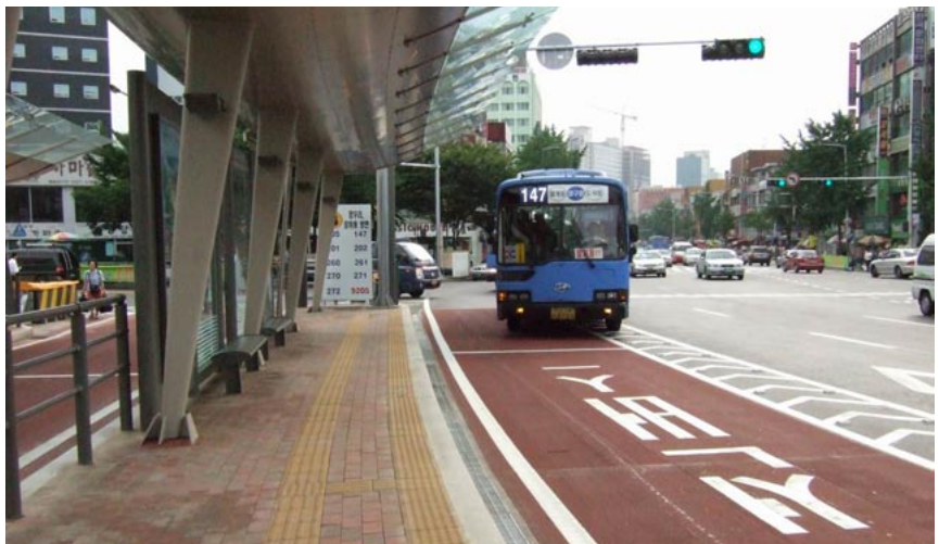
Figure 51 Reliability attracts more passengers. An exclusive bus lane like this one in Seoul improves travel time.
