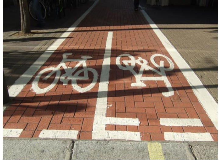
Figure 36 A well designed bicycle lane with painting and textured pavement in London.
