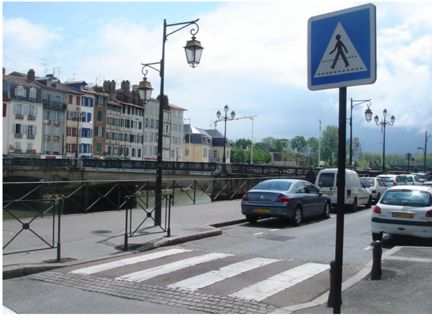
Figure 33 A roadway neckdown, sign, and speed bump ensures that cars slow down in Bayonne.
