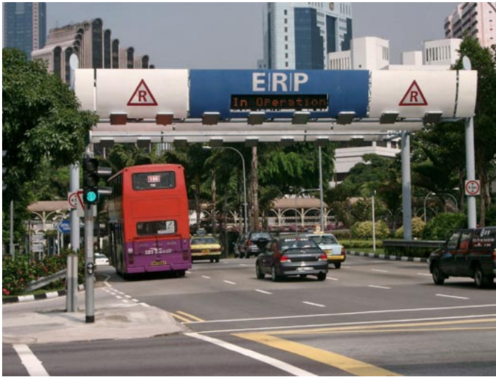
Figure 65 Singapore’s Electronic Road Pricing (ERP) gantry automatically deducts payment from CashCards inside In-vehicle Units (IUs).
