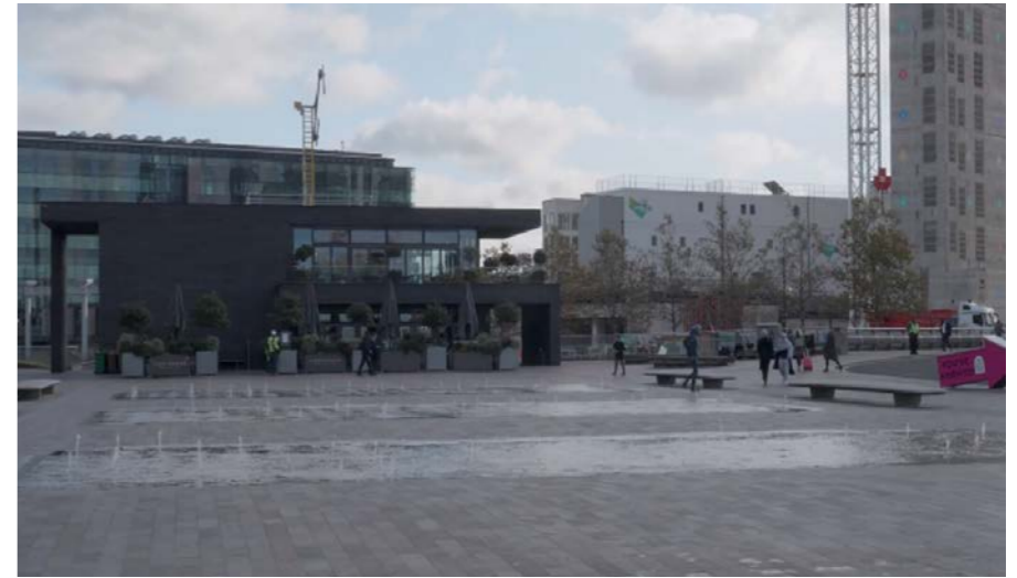
Figure 32: King's Cross station area after the redesign in London / United Kingdom (GIZ, UCL 2020)
