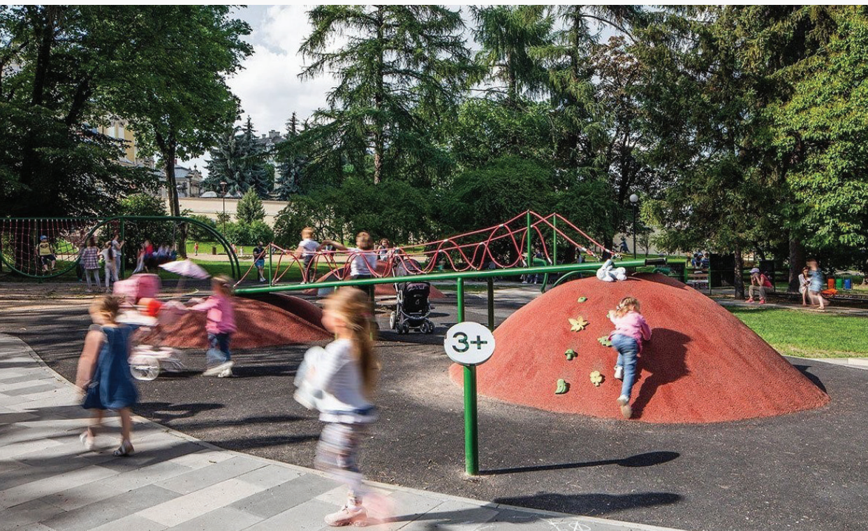
Newly constructed playground in Lviv. Source: TUMI.
