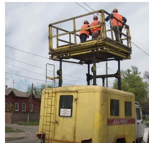
Repair of trolleybus catenary in Chernihiv (Source: Screenshot from: https://www.youtube.com )
