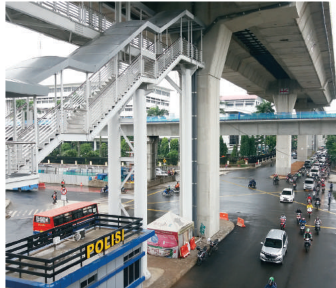
Top left: Transjakarta BRT Corridor 13, the first elevated BRT in the Jakarta transit system, opened in 2017.
