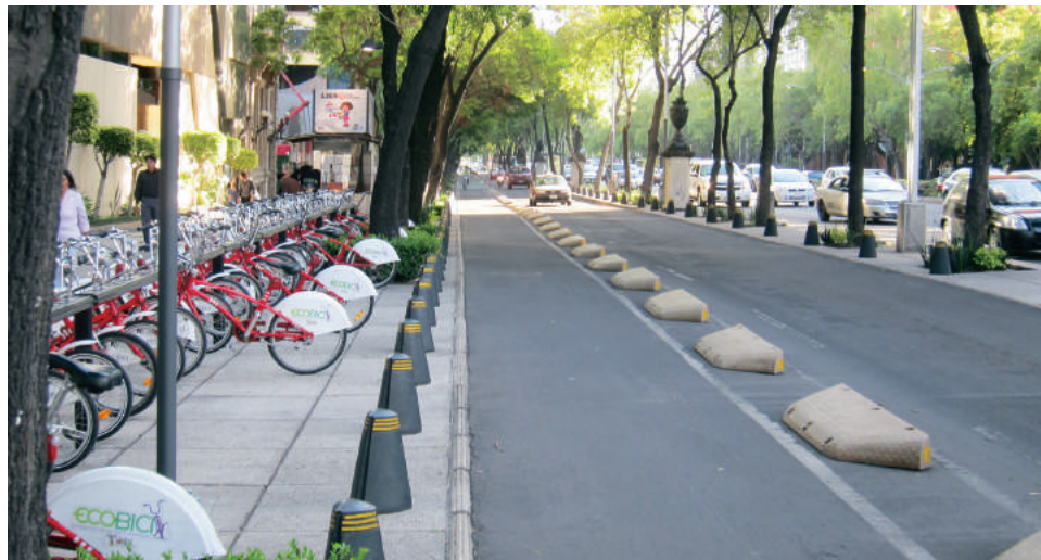
Pedestrian bump-outs, protected bike lanes, and road diets are just few design elements that Mexico City has implemented – in addition to eliminating parking minimums – to promote low-carbon walking and cycling.
