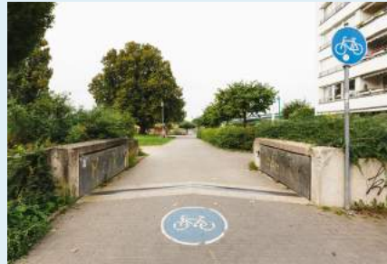
Figure 25: Did you spot the floodgates on the cycling paths?, photo by Philipp Böhme
