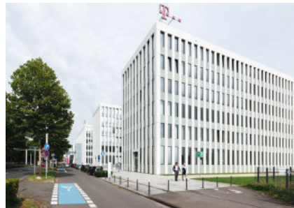
Figure 28: Friedrich Ebert Allee with Deutsche Telekom HQ (the car lanes are on the left side of the hedge), photo by Philipp Böhme
