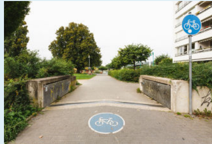
Figure 22: Did you spot the floodgates on the cycling paths?, photo by Philipp Böhme
