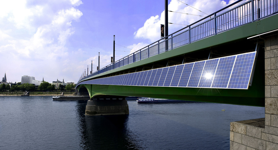
Figure 10: Solar panels on Kennedybrücke, photo by Nicole Funk
