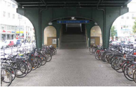
Figure 14: Intermodality: Bicycle parking at the entrance to a subway station © Sven Ledwoch
