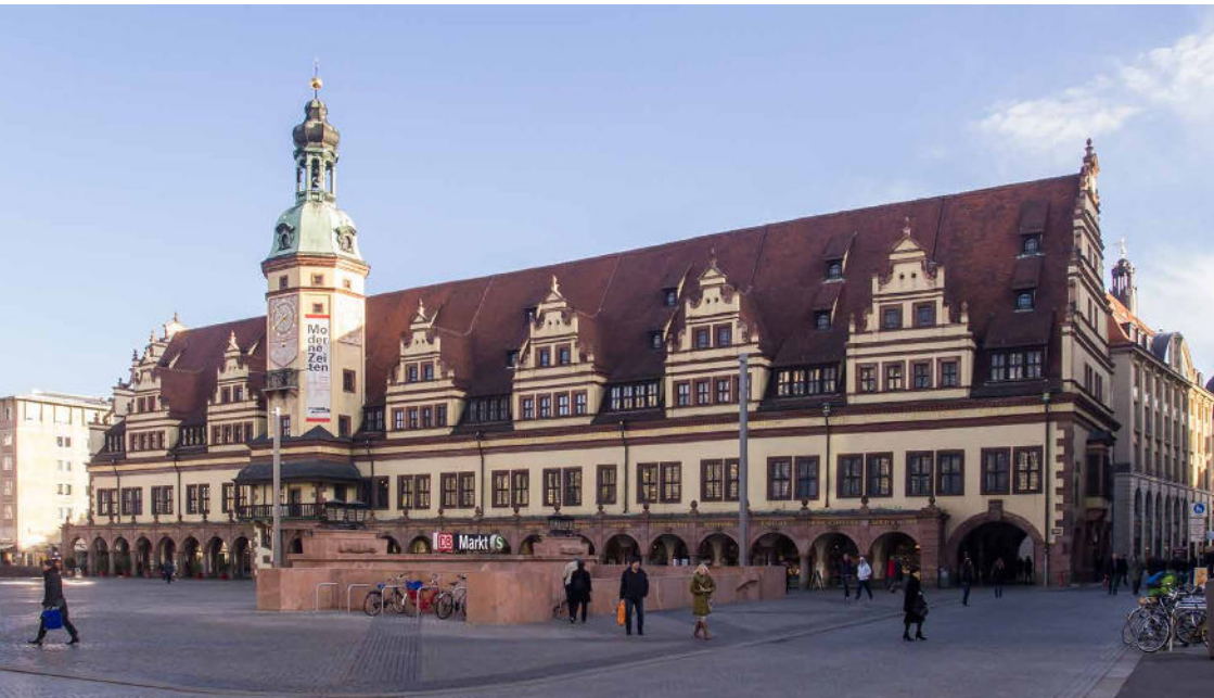
Figure 11: Entrance to the new market station; © Ed Webster on Flickr/ CC BY 2.0
