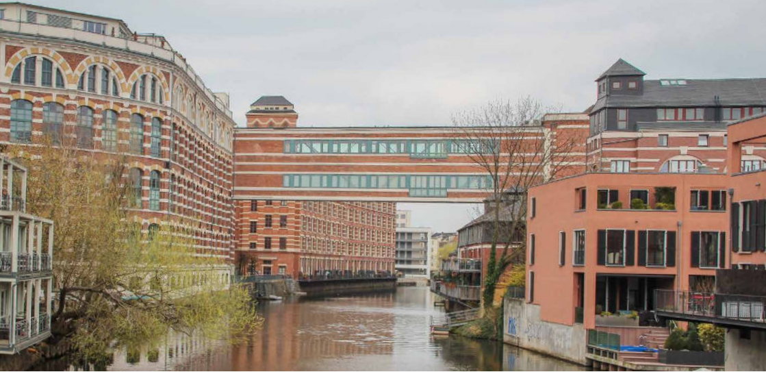
Figure 29: View from Karlbrücke; © Zoe Back
