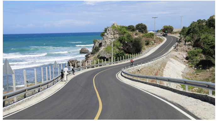
Source: It All Starts With a Road: The Key to Mobility in Haiti
