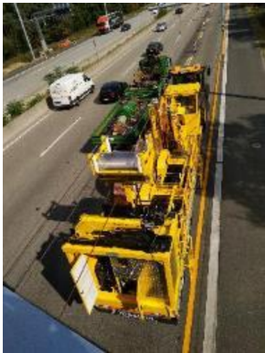
Pulling the contact line
