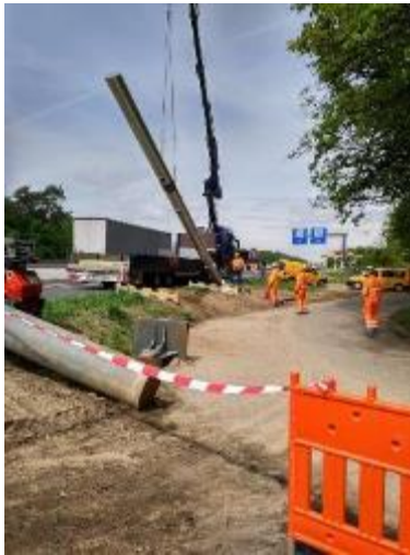
Erecting poles
