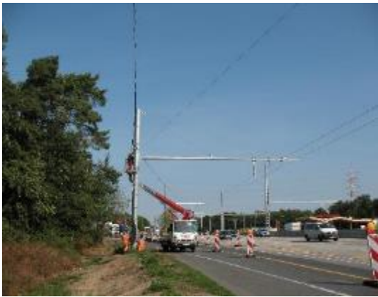
Attaching cantilevers
