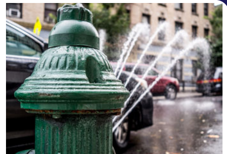
Fire hydrants © Phil Roeder, Wikicommons CC BY 2.0
