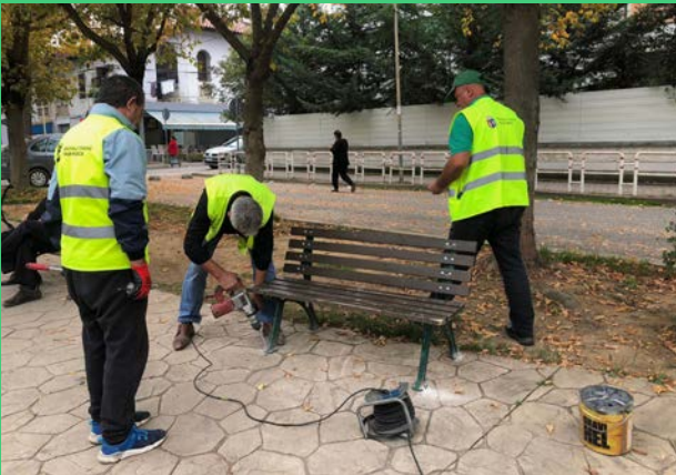
The maintenance department is pictured installing a new bench under the shade of a tree. Image credits: City workers' Twitter account.
