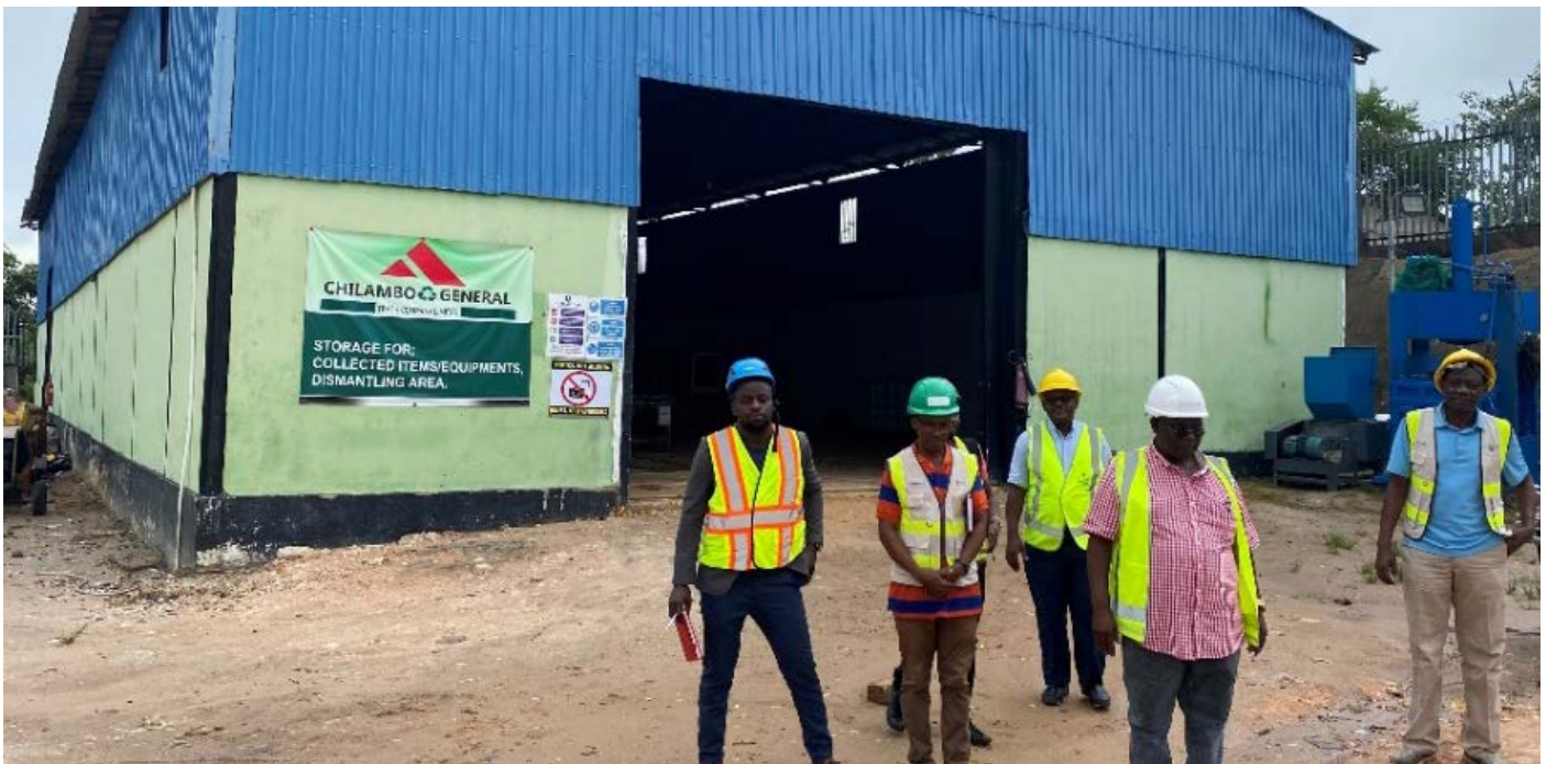
Figure 8. Storage and dismantling area of Chilambo General Trade Company Ltd. (Source: Oeko-Institut e.V.)
