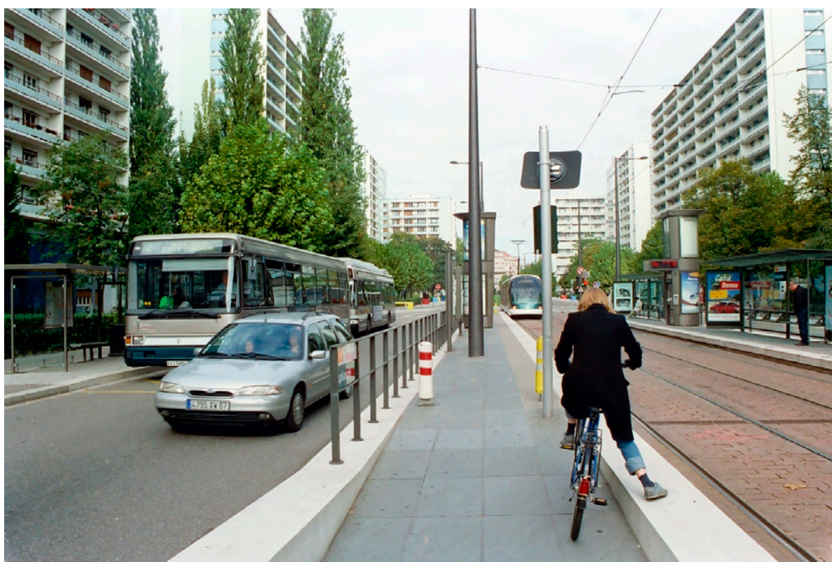
Figure 39: Light rail-bus station in Strasbourg. © Robin Hickman 2003
