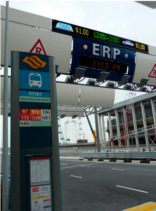
Figure 56: Electronic road pricing helps to control vehicle access Singapore's city centre. The generated revenue is partially used for public transport operations. © Manfred Breithaupt 2010
