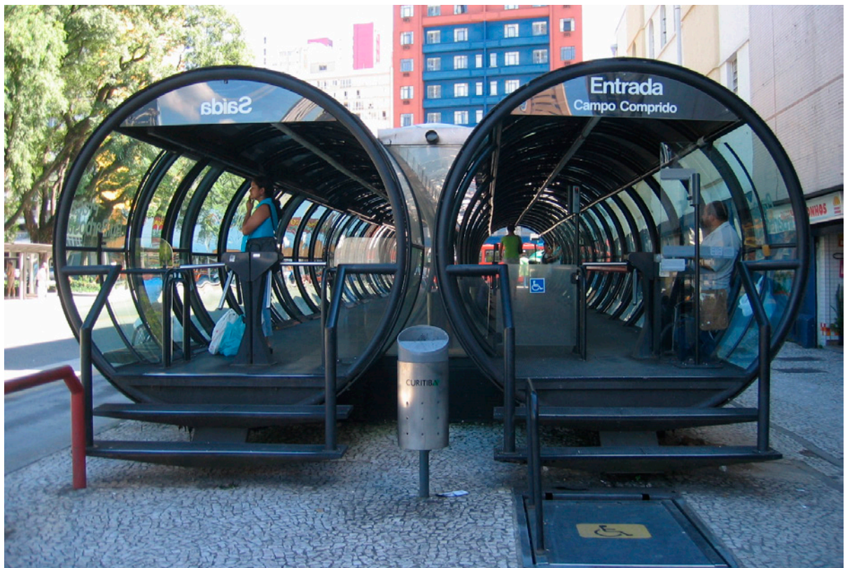
Figure 35: Elevated BRT station protects passengers from weather influences and contributes to safety aspects in Curitiba, Brazil. © Karl Otta 2005
