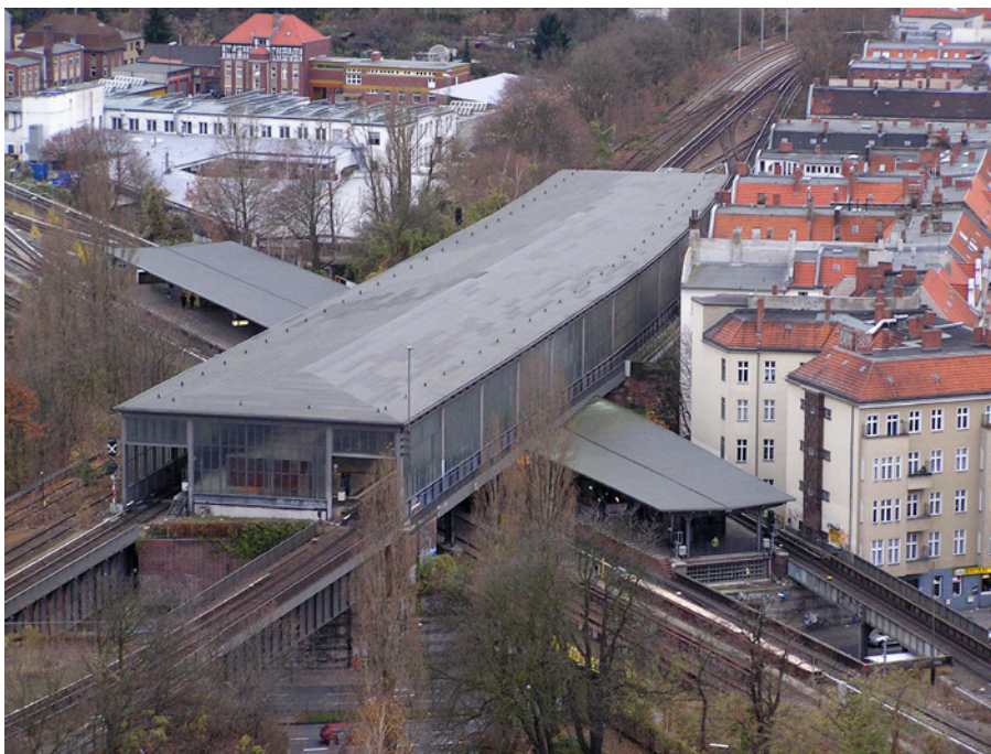
Figure 41: Multi level metro-metro station (Berlin Schöneberg). © Axel Mauruszat 2007
