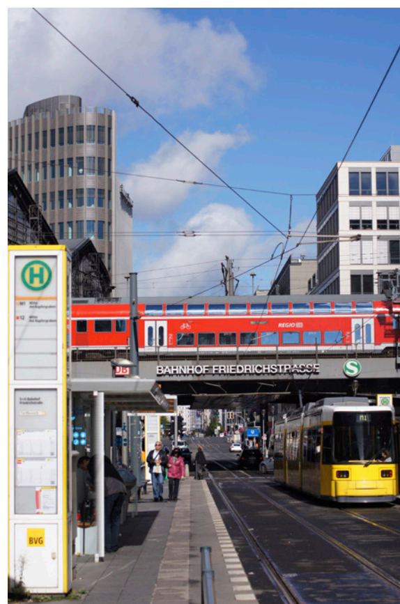
Figure 2: Interchange station between tram, bus, commuter rail (S-Bahn) and regional trains in Berlin.
