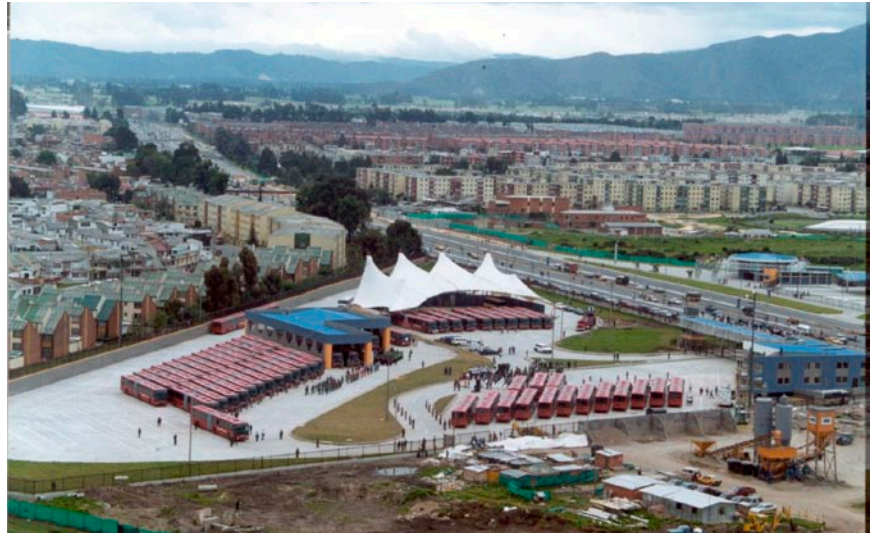
Fig. 62 Bus depot and maintenance area in Bogotá. Photo courtesy of TransMilenio SA.
