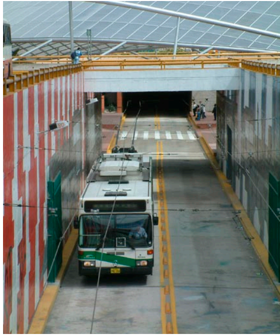
Fig. 46 and 47 Quito avoids conflicts at intersections by providing exclusive busway underpasses. The relatively modest cost of each underpass (US$ 1 million) is justified by the time savings achieved.
