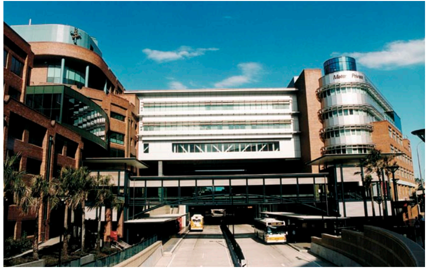
Fig. 41 In Brisbane (Australia), BRT vehicles have exclusive use of the entire roadway. Photo courtesy of Queensland Transport
