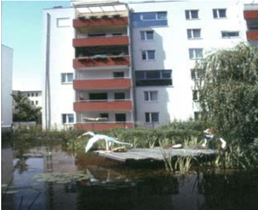
Fig. 64 The Floridsdorf car-free housing project in Vienna combines an aesthetically-pleasing environment with mixed-use planning to deliver a high-quality living experience.
