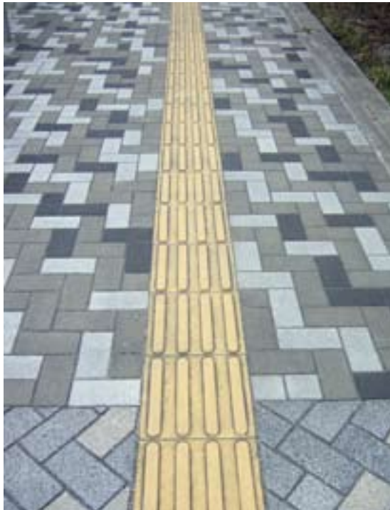
Fig. 172 Raised pavement markers provide invaluable guidance to sight-impaired persons. Photo by Lloyd Wright
