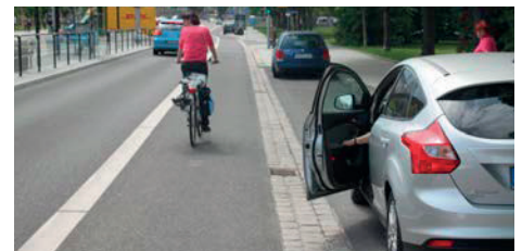
Sufficient safety clearance between parking lane and cycle lane (source: Tomas Cach)
