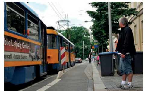
Elevated cycle lane at tram stop in Leipzig (source: Radka Žaková)
