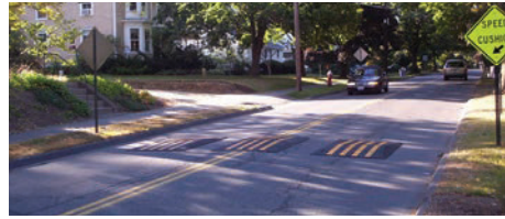
Figure 2: Speed humps leaving space for cyclists passing in the USA (Larry Kelley, onlyin-therepublicofamherst.blogspot.de)
