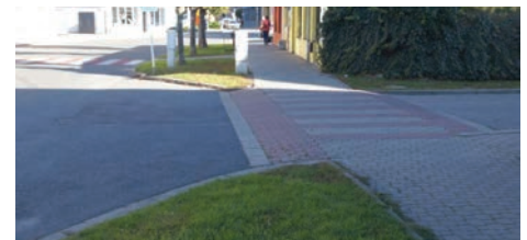
Figure 1: Elevated crossing in Uherské Hradiště (Jan Schubert)
