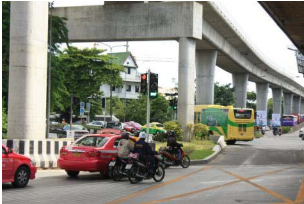
Figure 18: Signal Priority for BRT. There are 3 intersections where signal priority is given for the BRT.
