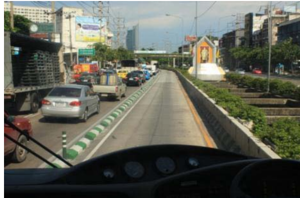
Figure 3: Physically segregated section of Bangkok BRT
