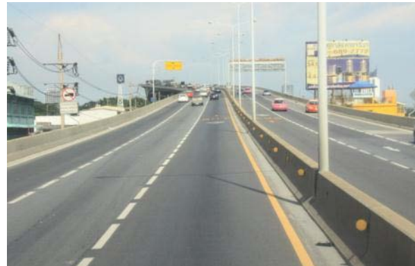
Figure 4: The BRT lane on one of the overpasses. The lane is also a High Occupancy Vehicle (HOV) lane
