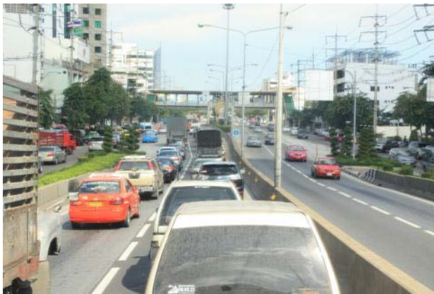
Figure 20: An unsegregated BRT lane congested with regular traffic. This shows that lack of segregation will hinder the smooth functioning of the BRT.
