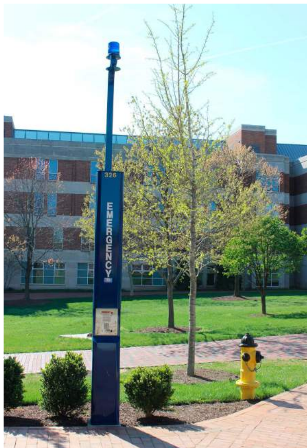
Fig. 6 : Emergency call box at University of Maryland campus (KORFFMANN 2016)
