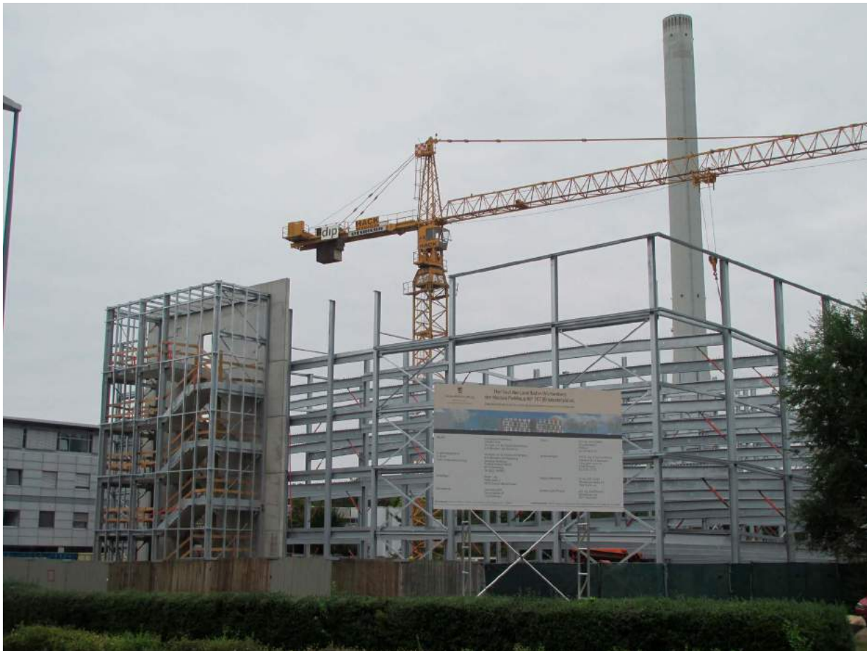
Fig. 5 : Construction of parking structure in Heidelberg next to Berliner Straße (KORFFMANN 2016)
