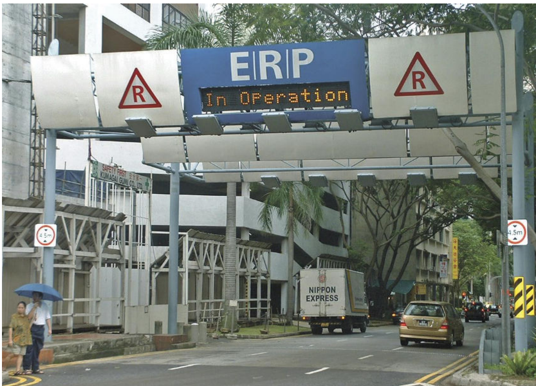
Fig. 9 The Singapore Electronic Road Pricing gantries impose charges on private vehicles entering the central area.
