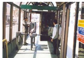
Fig. 27 BRT station in Quito, Ecuador: US$35,000
