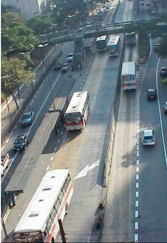
Fig. 5 Sao Paulo has the world's most extensive bus lane network, with 28 km of median busways and 137 km of bus lanes.
