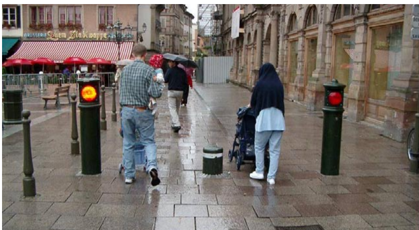
Figure 5 Concealable barrier for cars at the entrance to a car free zone, Strasbourg. Source: GTZ 2003
