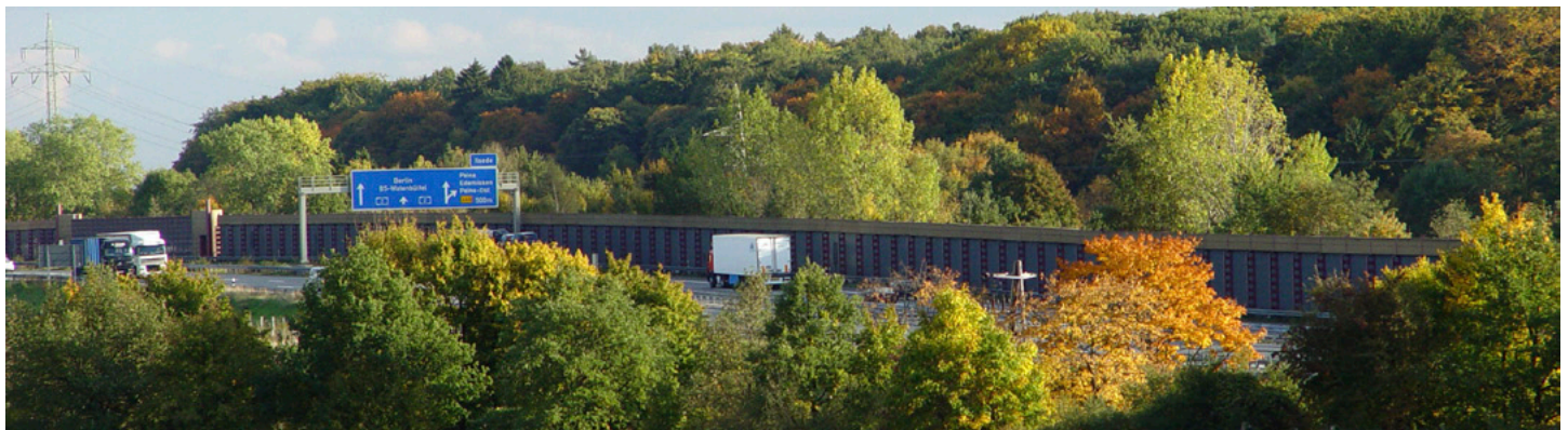
Fig. 23 A reasonable implanted noise barrier protects a near-by recreation-forest-area from the heavy noise emitted by the never-ending stream of cars and trucks on a highway in Germany. Klaus Neumann, 2009
