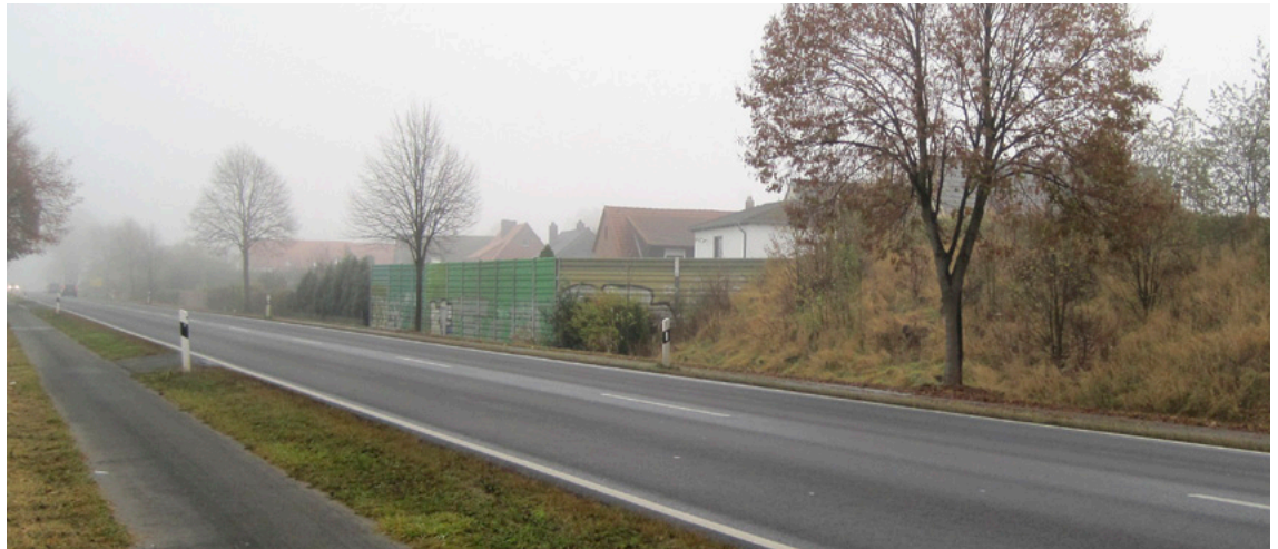
Fig. 22 Noise barriers designed as wooden or concrete walls (center of the photo) occupy less space than a heap-up earth wall (right side of the photo). Klaus Neumann, 2011
