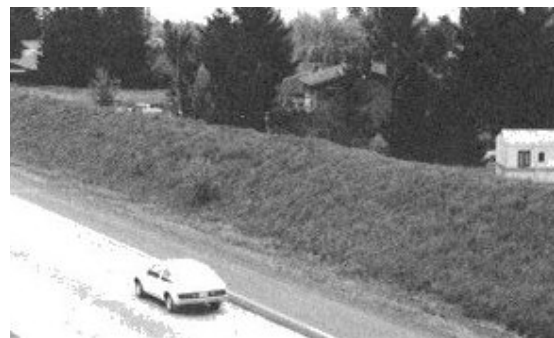
Earth Berm Noise Barrier
