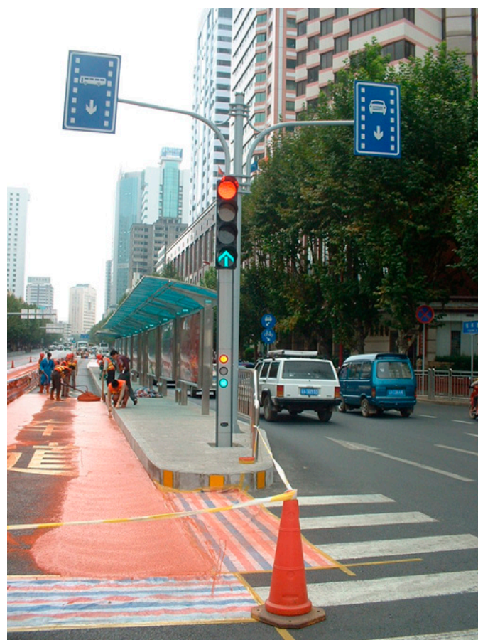
Figure 30: The BRT in Kunming: BRT lanes are being painted red. © Karl Fjellstrom, Kunming, 2003
