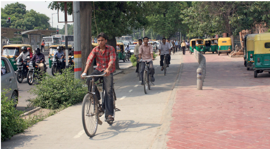
Figure 17 Bicycle tracks run parallel to the BRT corridor in Delhi.
