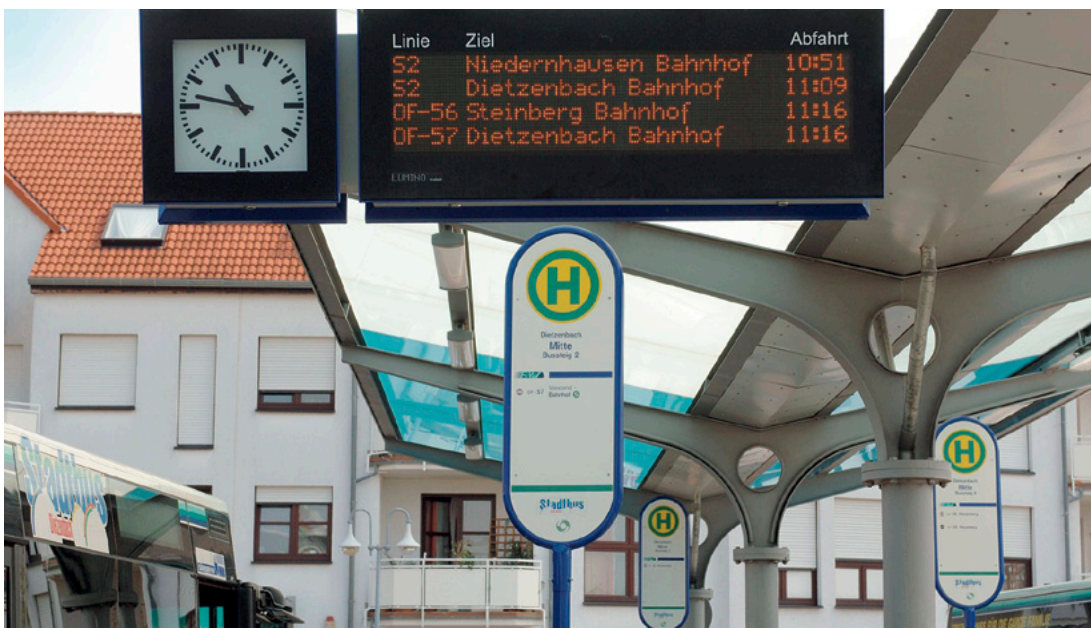
Figure 43 Dynamic passenger display system in use within the Rhein-Main-Verkehrsverbund (RMV).
