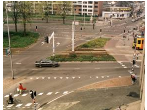
Intersection in Utrecht , Netherlands , where each mode (foot, bike, car, trolley) has its own lane and signal.
