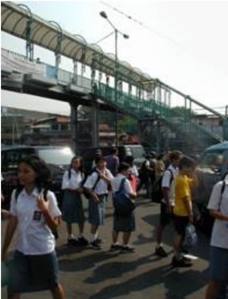
A needlessly high pedestrian overpass with steep steps in Jakarta is under-utilized and ineffective
