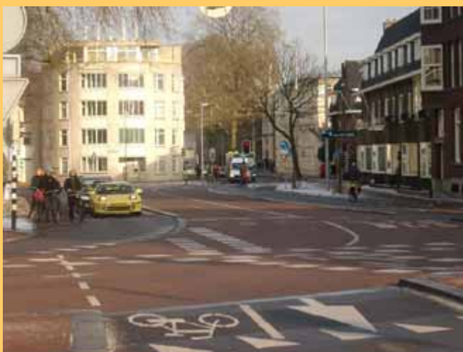
Separate bus and bicycle lanes through an intersection in Utrecht, The Netherlands. Roelof Wittink, I-ce
