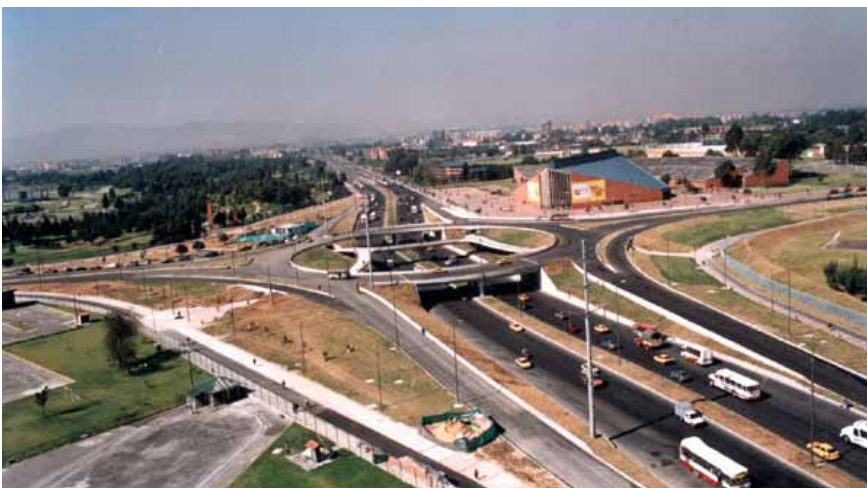
Bogotá: North-South motorised traffic elevated, East-West motorised traffic depressed, and facilities for non-motorised travel are at ground level.
