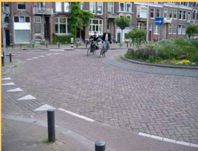
Mini roundabouts lower speed and facilitate safe integration between cars and cyclists (Utrecht, The Netherlands). Roelof Wittink, I-ce
