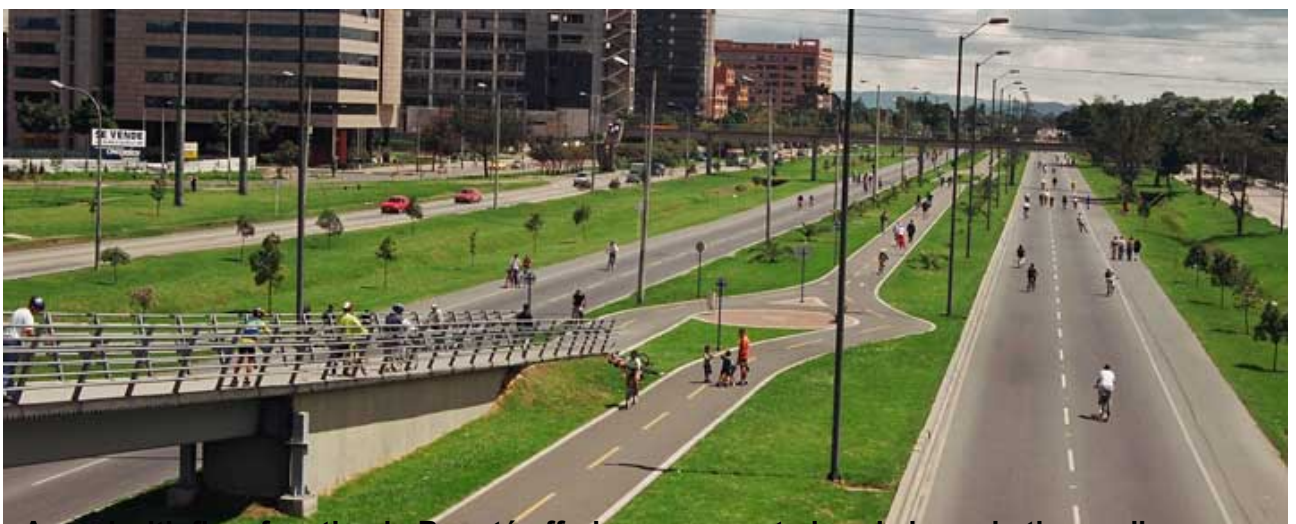
A road with flow-function in Bogotá offering segregated cycle lanes in the median strip - Photo taken during Ciclovía (car free sunday)
