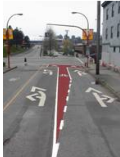
Bike Box (orients cyclists to bike lane on bridge), Vancouver BC , Canada
