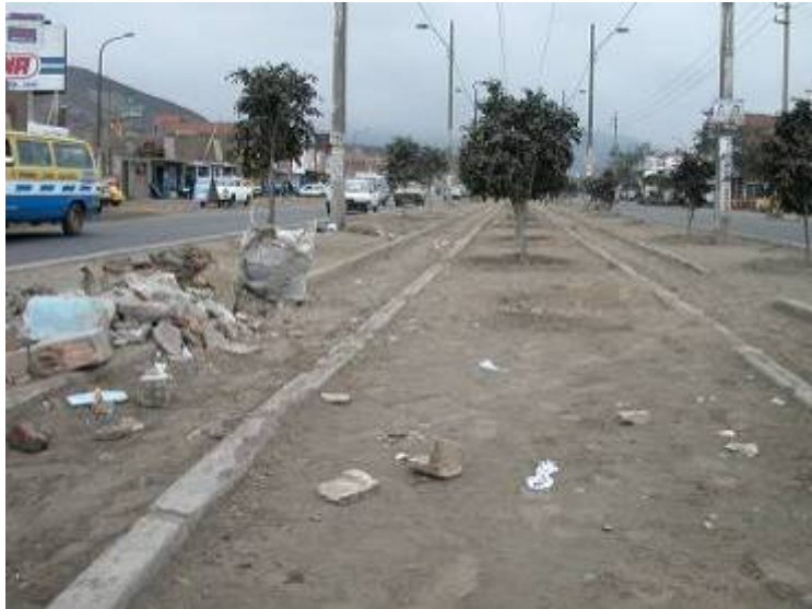
Figure 8. The photo above presents the bikeways of Lima (Peru), 8 years after their construction in 1994. The lack of a clear promotional strategy in 1994 made it unlikely that the public would use the bikeways, despite the presence of adequate infrastructure in the beginning. The photo shows how the bikeways have been covered in dust because of lack of use (and maintenance). Source: Fundación Ciudad Humana, GTZ Transport Photo CD.
