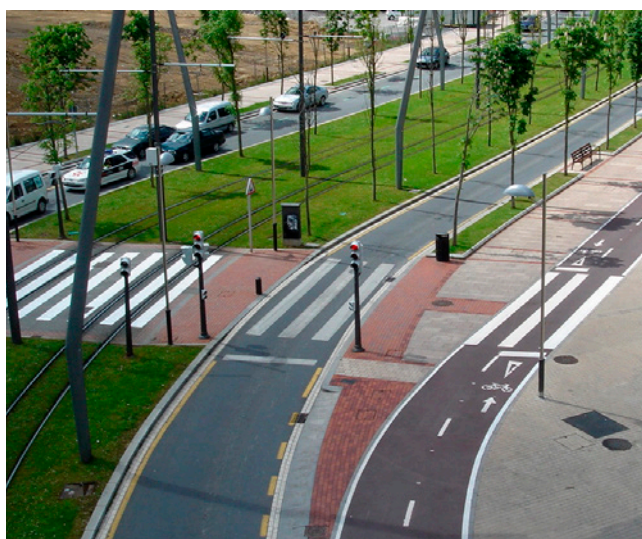
Figure 11: Four Modes, four different lanes – Mode separation for light rail, motorised traffic, cyclists and pedestrians. © Andrea Broadous, Bilbao, Spain, 2008
