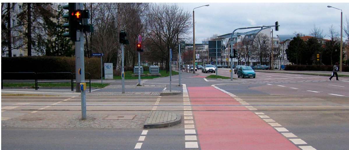
Figure 14: Cycle paths marked red on intersections raise driver’s attention for non-motorised traffic.
