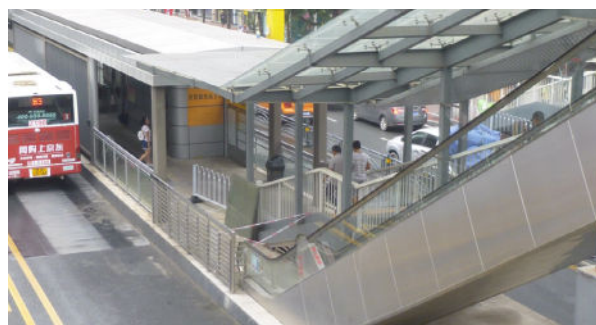
Figure 12: Escalators not working at a BRT station. Photo by Heather Allen.
