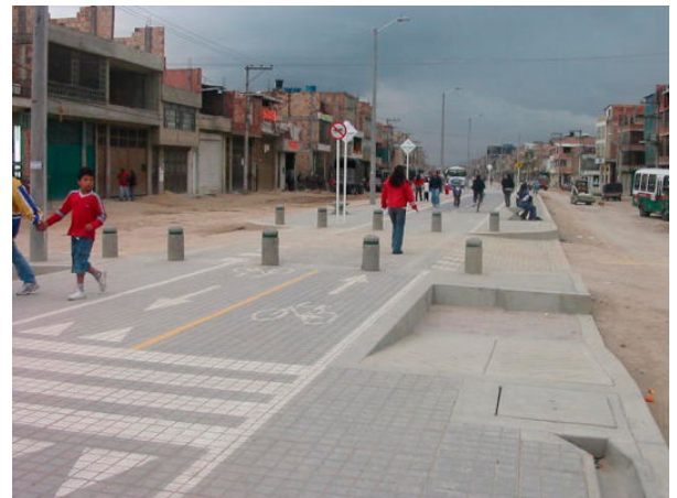
Figure 37: Alamedas in Bogotá were built on the side of dusty roads, showing that pedestrians were more important than automobiles. Source: Por el País que Queremos.
