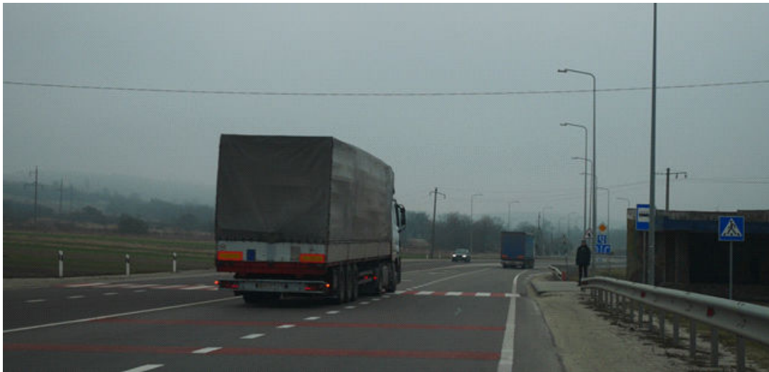
| International road of national significance and a zebra crossing
