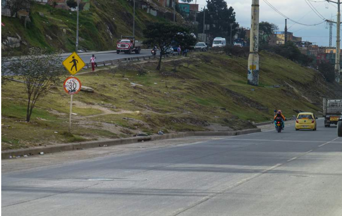
Figure 3. Poor coordination between the speed limit and the infrastructure. Photo: Natalia Lleras
