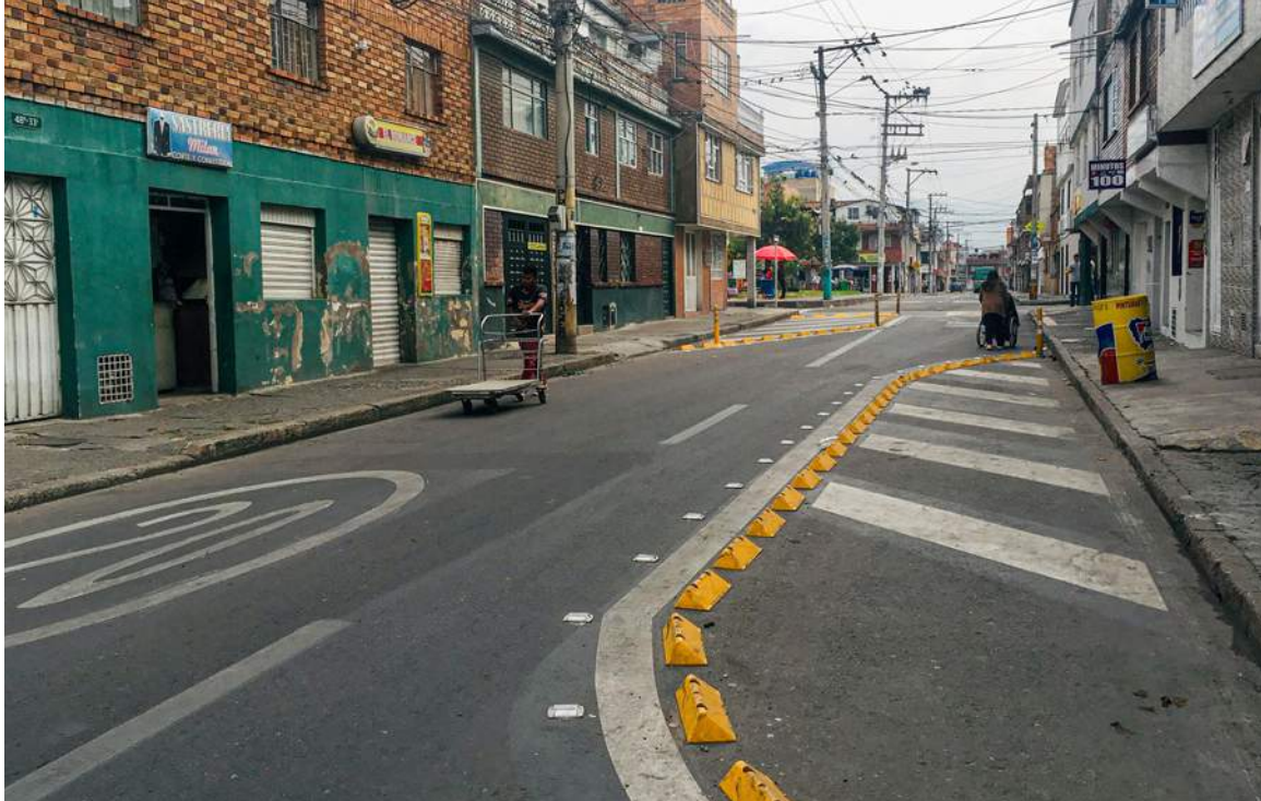
Figure 4. Traffic calming measures implemented for speed limit compliance in Bogota. Photo: Natalia Lleras
